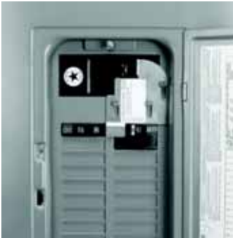
Cutaway Showing Installed Generator Interlock Kit
