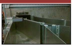
Exlar's Tritex II actuator installed on one of Portland General Electric's fish diverter doors.
