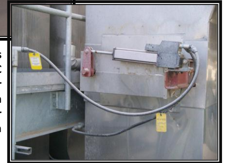
After: Exlar's Tritex II AC actuator installed on damper application
