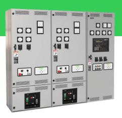
From two-generator prime power to redundant 22-generator mission-critical facilities, ASCO Power Control Systems manage and optimize multiple power sources and downstream loads.
